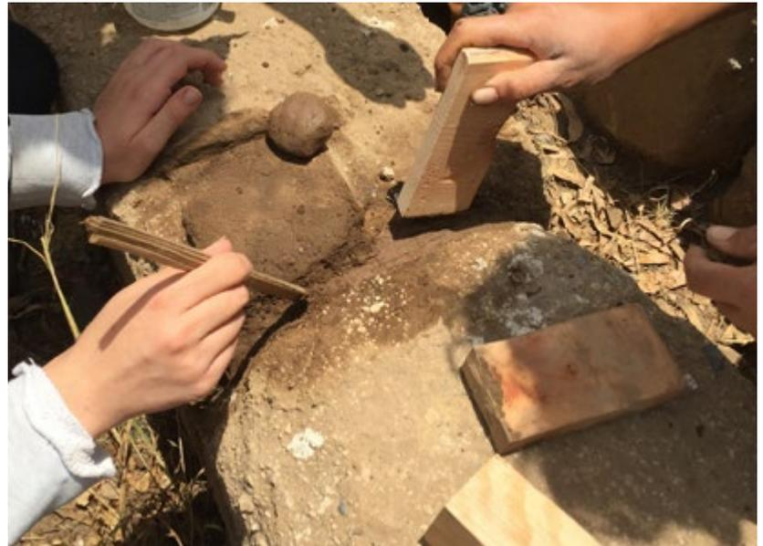
If the damage to the walls is very deep, such as in continuous fissures or cracks, equidistant tubular “nozzles” can be inserted over the entire length during the filling and compacting process. Once the closing of the crack is completed, a fluid clay paste stabilized with 5 to 10% in volume of calcium hydroxide is injected, which will be gravitationally distributed within the cores. Finally, the nozzles are extracted or cut away and the operation is completely sealed.
