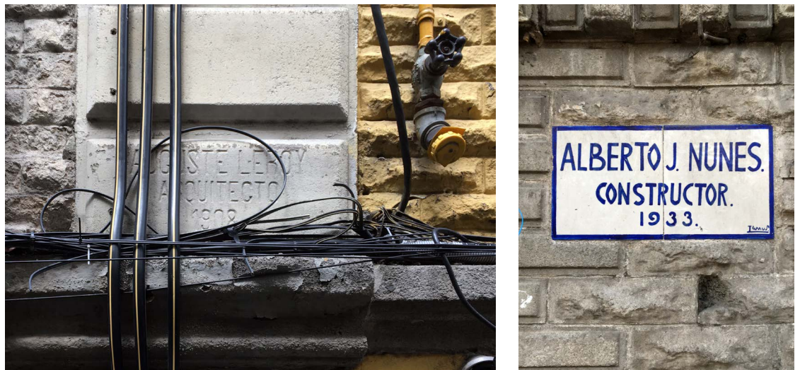
FIGURE 8. The dates of these two photographs comprise the first and last dates found in the field (in 2021) that verify the use of cement partition walls in Mexico City. Left, authorship signature of architect Auguste Leroy dated 1908; right, authorship plaque of builder Alberto J. Nunes dated 1933 (Photographs: Alejandro Leal & Alberto Muciño, 2021; source: Authors' Collection).
