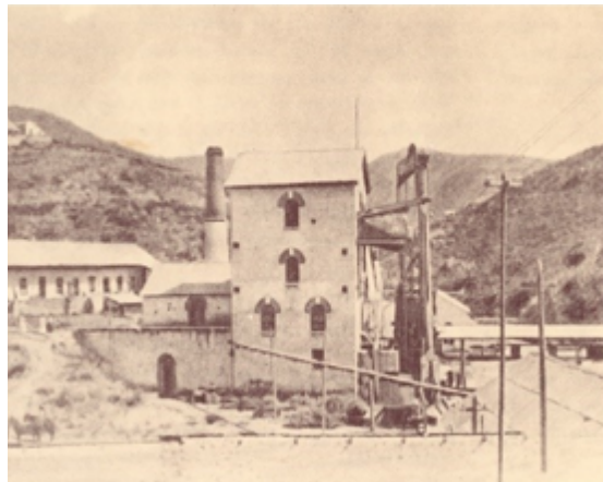
FIGURE 3. Maravillas Mine (Source: Soto, 1985, p. 250).
