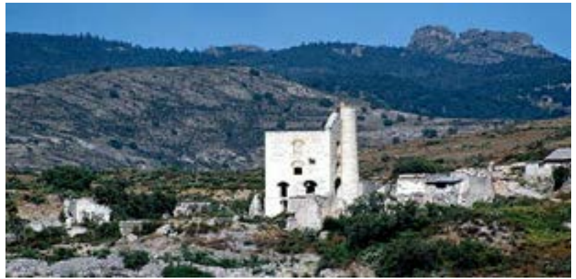
FIGURE 8. San Pedro la Rabia Mine (Source: Schwartz, 2021, https://projects.exeter.ac.uk/cornishlatin/cornishlatinamerica.htm )
